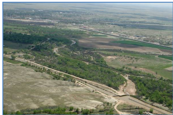
Fort Lyons Intake Canal Diversion Structure Photo by Dick Stenzel
